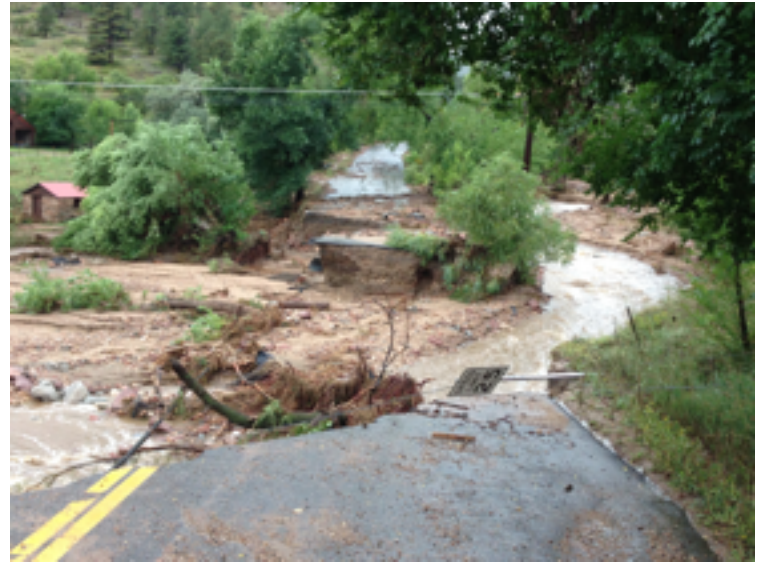
Erosion of Wagon Wheel Gap road
