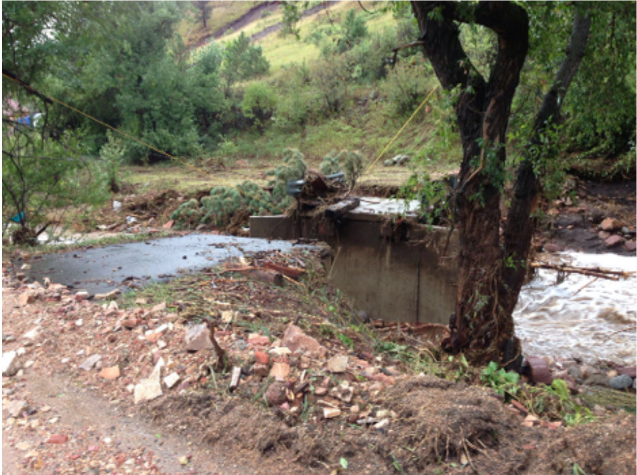
Bridge destroyed at “choke point” along Lee Hill Drive. Note the vegetation on the bridge deck indicating how high the flow was here (photograph taken September 15, 2013 by James V. Holmes).
